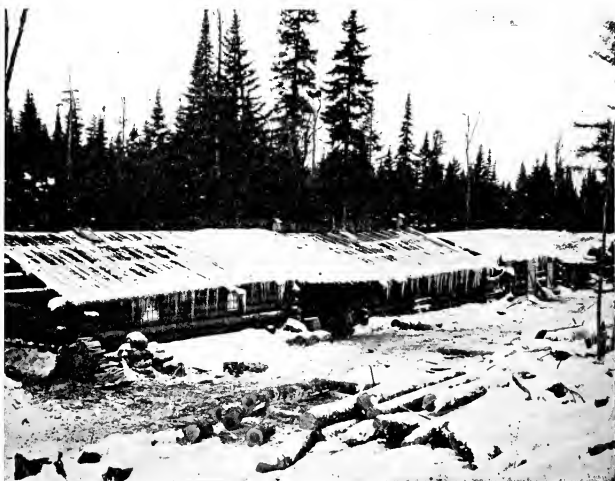
FIG. 2. — A Logging Camp in the Northeast. The buildings from left to right are the cook shanty, bunk house, blacksmith shop, and stable. Maine.
